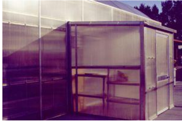
Figure 6. Vestibules at all entries help prevent insect entry.
