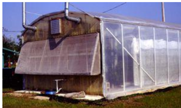
Figure 5. Fine mesh screening over all openings prevents insect entry.
