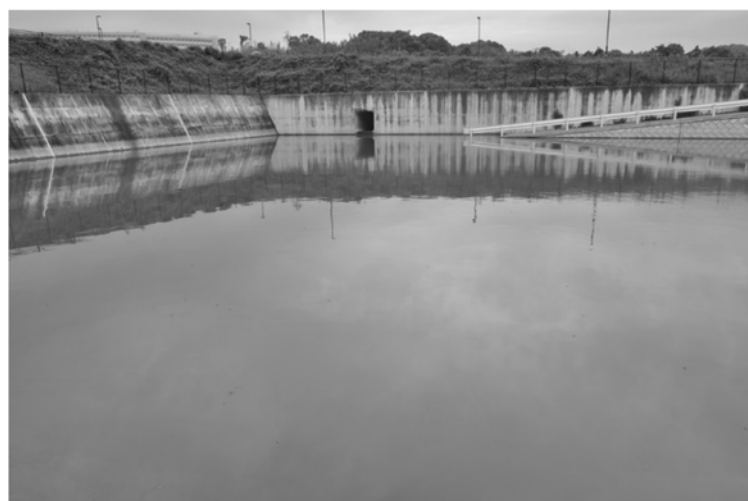
Fig. 2 Overall view of Pond A on May 29, 2018.
